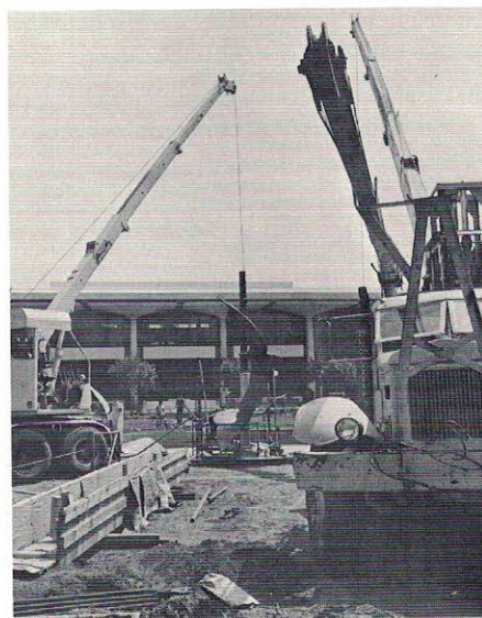
Number two bird hoisted into place.
